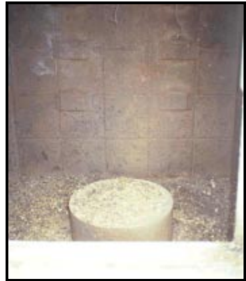
Interior view of the floor of a Donovan Blast Chamber.
