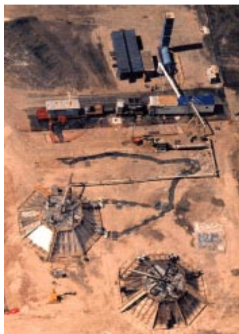
In-situ vitrification hoods.
